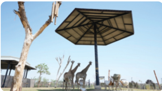
As part of summer management in the Herbivore area, shade structures were constructed to provide relief from the heat, enhancing animal comfort and promoting welfare during elevated temperatures.
